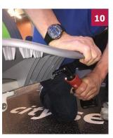
Maintain downward pressure on the front of the seat and tighten the bolts.
