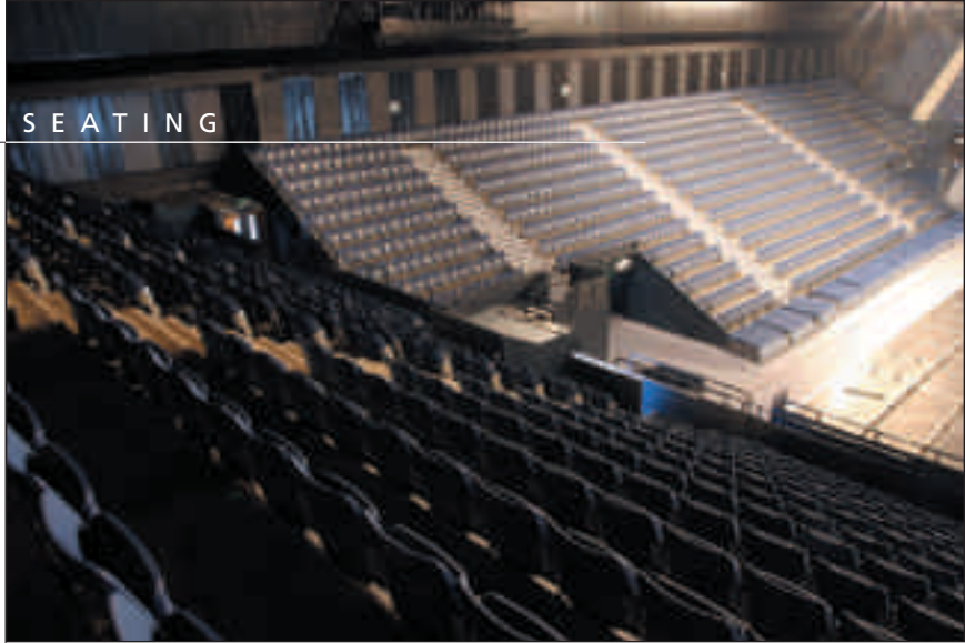
Audience Systems' refurbishment of Wembley Arena includes the fixed seating (foreground), removable matrix seating stacked up (in the centre) and the low rise retractable platforms (to the right).
